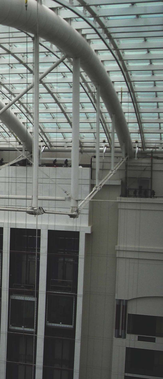
opposite: The 19-story atrium is topped with a 2,400-ton steel bow-string truss roof skylight structure.
