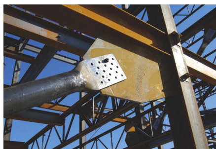
Figure 6: Installed Cast ConneX brace.
