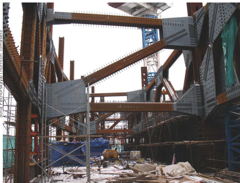
The west section of the 33rd-floor outrigger trusses, linking the belt truss on the left to the central core on the right.
