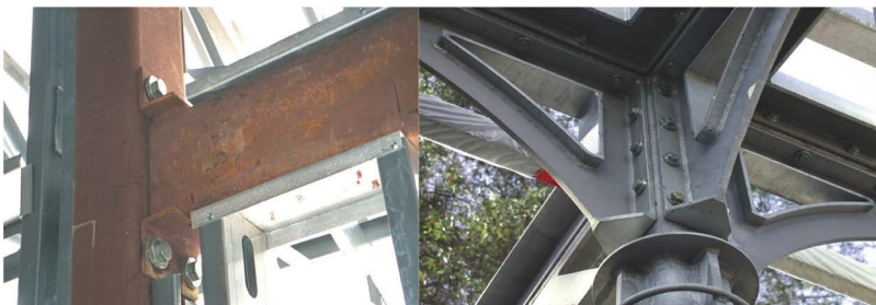
Figure 4: Picture of Hollo Bolt connection details.
